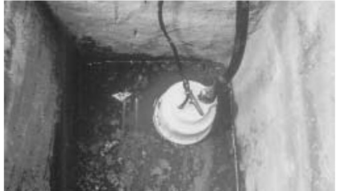
Figure 5.5. If the basement has a sump pump, care should be taken to avoid getting chemical into the “sump” or pit in which the pump sits. This is important because sump pumps usually discharge into non-target areas, such as a driveway, street gutter, or underground sewer.
