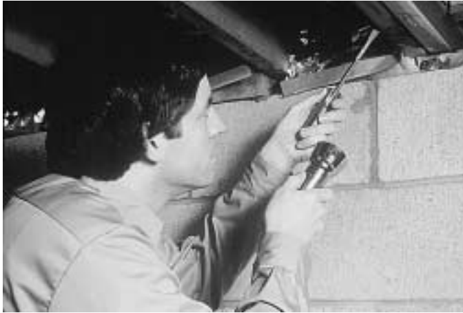
Figure 3.13. Probing the wood with a tool can help detect cavities.
