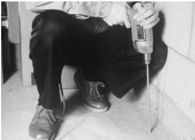
Figure 3.5. Slabs are drilled so that termiticide can be injected through holes to treat the soil beneath.
