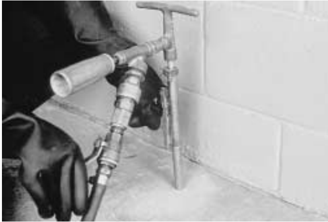
Figure 3.4 A slab injector used to inject termiticide under pressure into an area beneath a slab.
