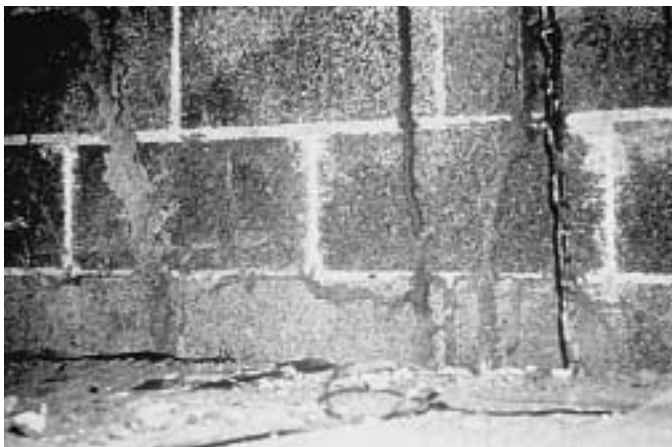
Figure 3.11. To reach wood in buildings, termite workers often make mud tubes up the outside or inside of foundation walls. These tubes protect the workers from natural enemies and help provide the moist environment they need.
