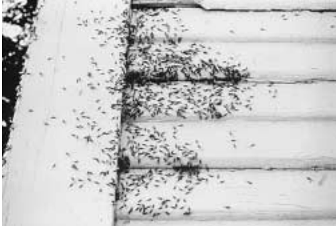
Figure 3.10. The presence of swarmers is often detected by the homeowner as the first sign of termite infestation.
