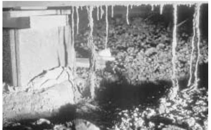
Figure 2.14. Free-standing shelter tubes.
